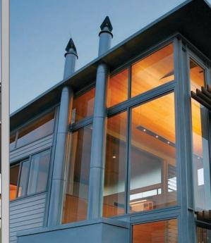
Directional bird cowls are designed to shift position in relation to wind direction as the wind turns the cowl in the opposite direction of the prevailing wind.
