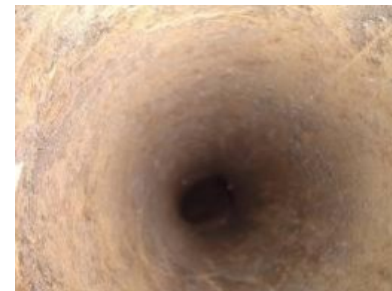
dia 1. Flue prior to cleaning
