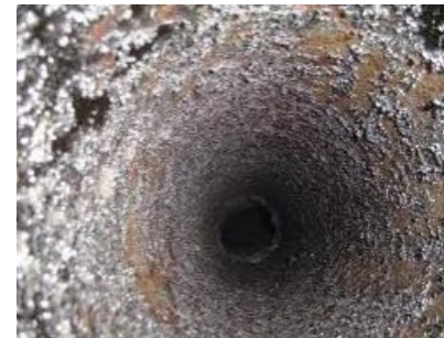
dia 1. Flue prior to cleaning
