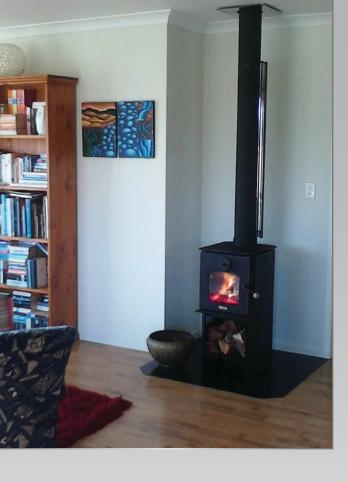
Floor protectors are required when installing a free-standing fire onto any combustible surface.
